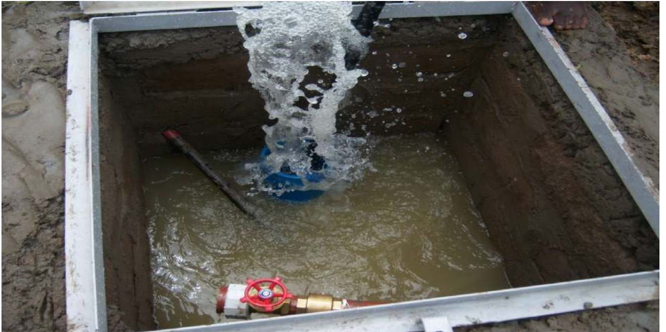
2 nd site water after 120meters we got water 2013
